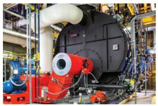
Low NOx by flue gas recirculation can be achieved by one of two methods either forced FGR or induced FGR, depending on application. Forced FGR is accomplished by forcing the flue gases with a separate fan back
