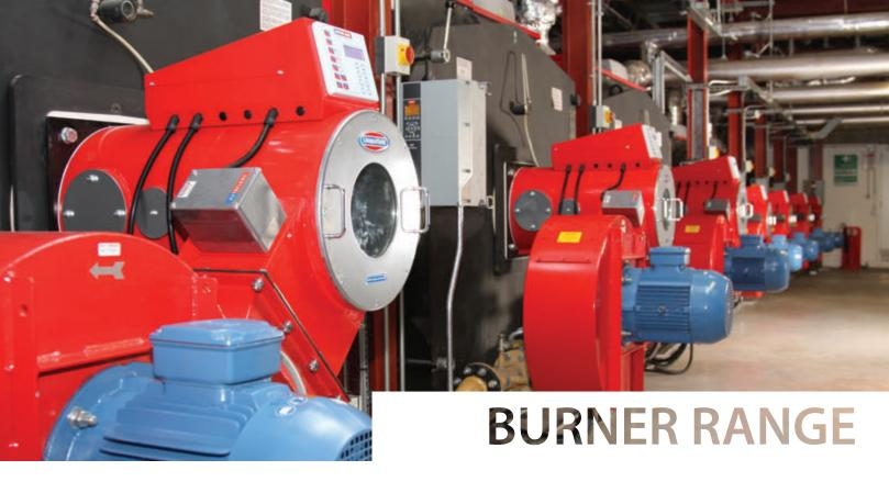
Limpsfield Combustion offer standard burners from 3,000,000 Btu/hr (0.9 MW) to 220,000,000 Btu/hr (62 MW), firing a wide range of fuels from natural gas, diesel, #2 oil to heavy fuel oil, waste oils, animal fats, fish oils, bio gases etc. Excellent results have been achieved when firing such fuels offering the end user substantial fuel savings through high performance.
