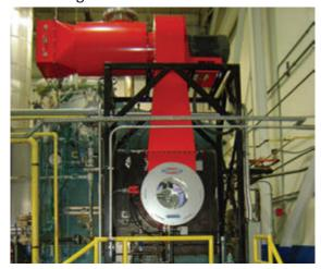
It is recommended that the pressure drop in the air duct between the outlet of the blower and inlet to the burner be no more than  $\frac{1}{2}$ " WC.
