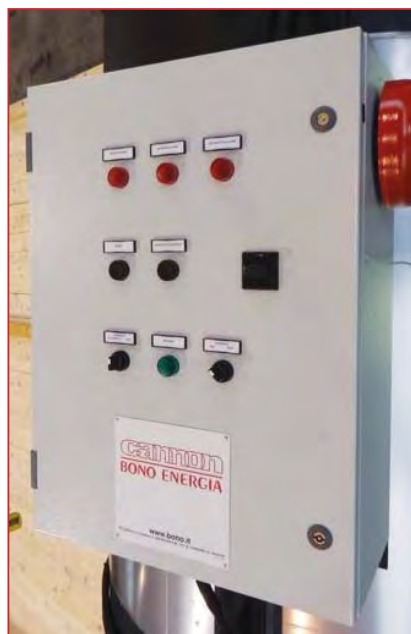
Figure 5 Control panel for UNI-MATIC UM steam generator.
